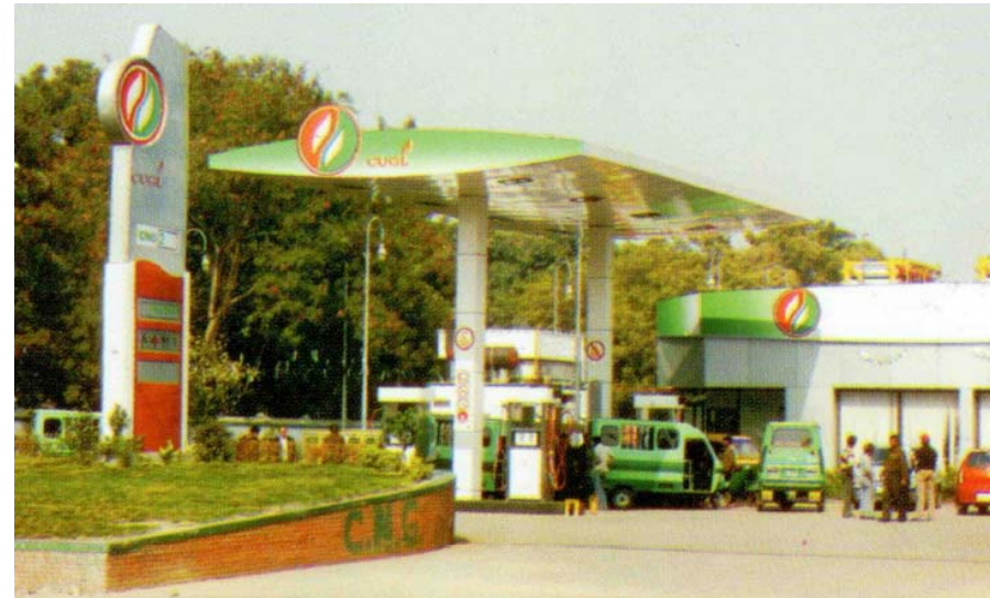
Fully Operational CNG Station of the Company at Fazalgunz, Kanpur
