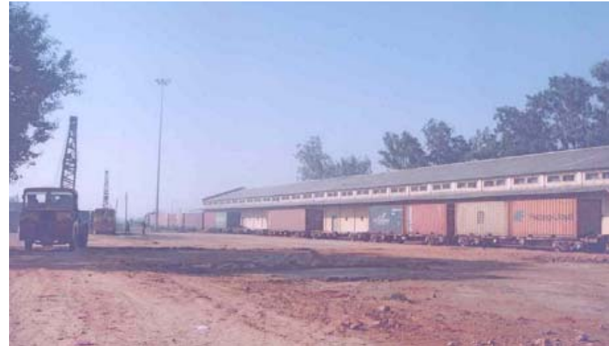
Inland Container Depot Under Development at Loni, Delhi
